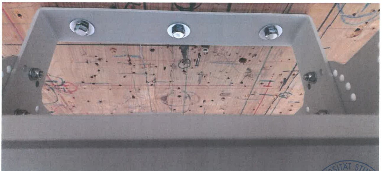
Figure 2 Detail: suspension of the installation element "SPACE-2".
